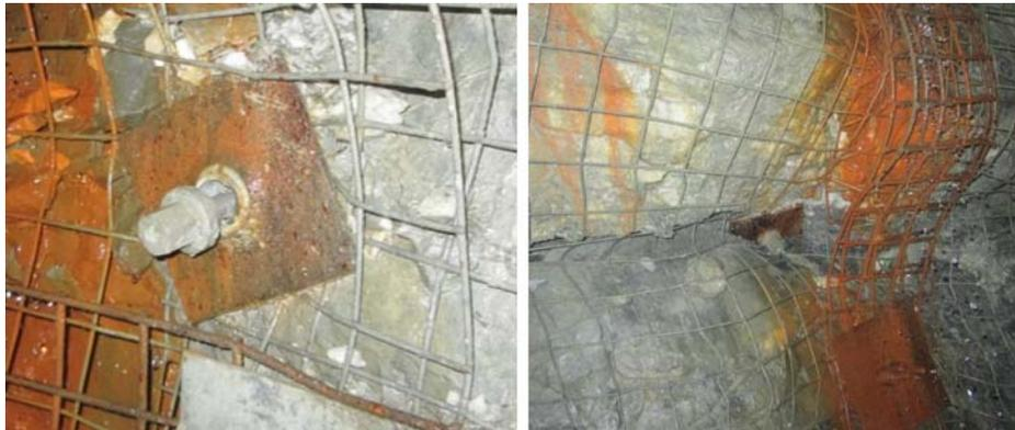
FIG 7 – Combination bolt failure – tensile failure on the left, shear on the right
