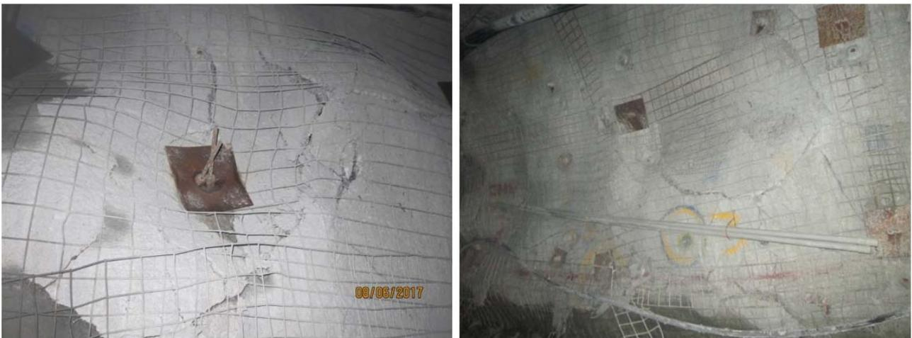
FIG 5 – Failed fibrecrete due to ground movement
