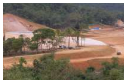
Plant Site Investigation/Design (Indonesia)
